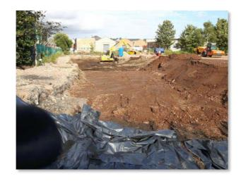
Dunton Environmental Ltd was appointed by G F Tomlinson Buildng Ltd in July 2016 to carry out shallow earthworks, remediation and verification testing prior to development of a new Advanced Manufacturing Building, located in the southern part of the Jubilee Campus Extension of the University of Nottingham, Derby road in Nottingham.
