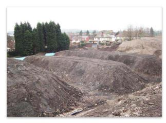
After treatment, the soils were tested and placed in a stockpile on site pending validation. On successful validation of all the soils, they were **re-used on site** in accordance with the agreed requirements.
